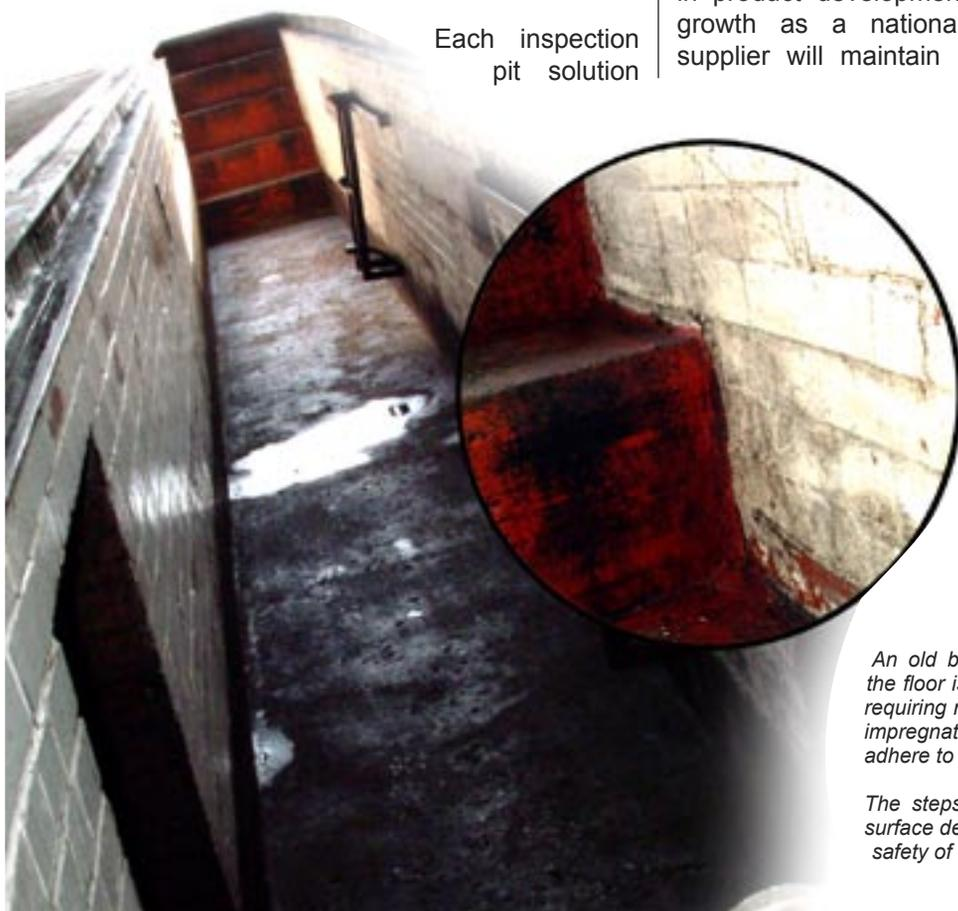
An old brick pit with concrete floor. Note how the floor is damp and that the gloss paint finish is requiring maintenance. Once oil and grease have impregnated the brickwork, no amount of paint will adhere to the pit walls.
